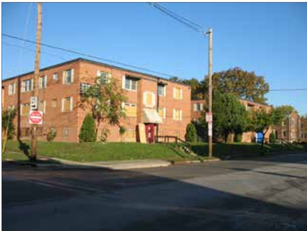
Two apartment buildings located on the corner of North Fourth Street and East Eighth Avenue were magnets for crime and have been demolished.
