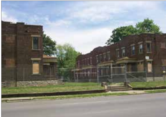
CPO apartments under renovation
