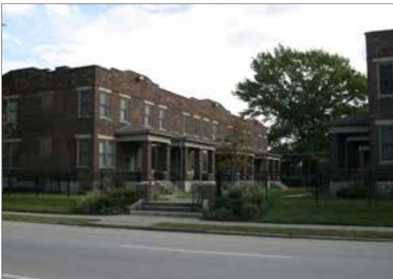
CPO completed renovations
