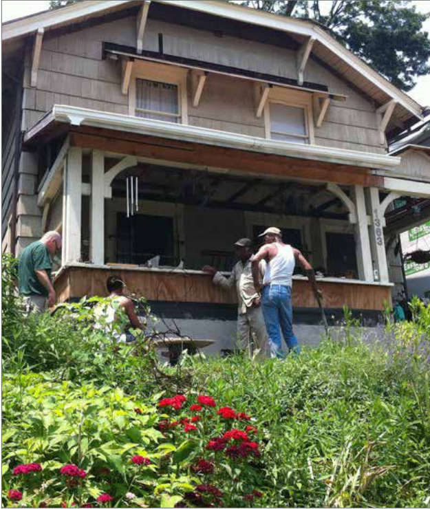
The Exterior Home Repair Program assists homeowners with needed renovation work.
