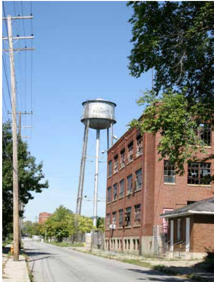
Campus Partners, the City of Columbus, and Wagenbrenner Development cooperated on the demolition and clean-up of the former Columbus Coated Fabrics site.
