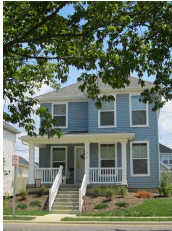
New homes constructed with Low-Income Housing Tax Credits provided a lease-to-purchase option in the neighborhood.
