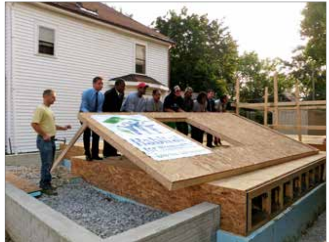
Habitat for Humanity wall raising, August 2011
